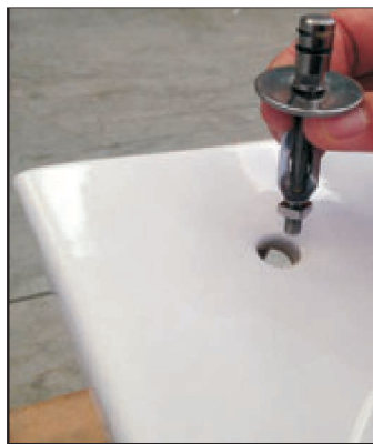
02 Vložit úchyt do otvoru WC. Insert the screw in the appropriate hole.
